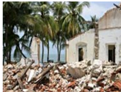
Back view of the house, demolished courtyard. Photo © Jim Rosenberg.
